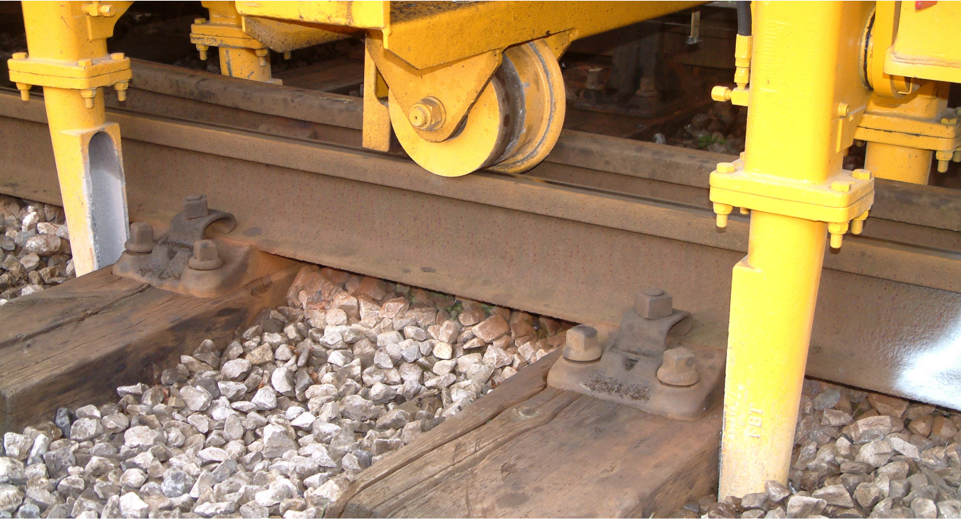
Multipurpose Stoneblower injecting stone under sleepers to lift track
